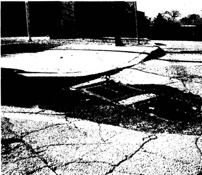
Figure 3 – Ramp in poor condition at the entrance of Rouge Valley Health Center
